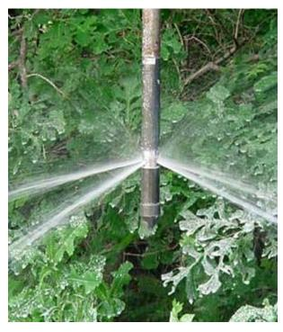
distribution of slurry over the targeted depth interval. At the end of each injection point, a small volume of water (15 USG) is often used to clear the rods and the injection tip of any slurry.
