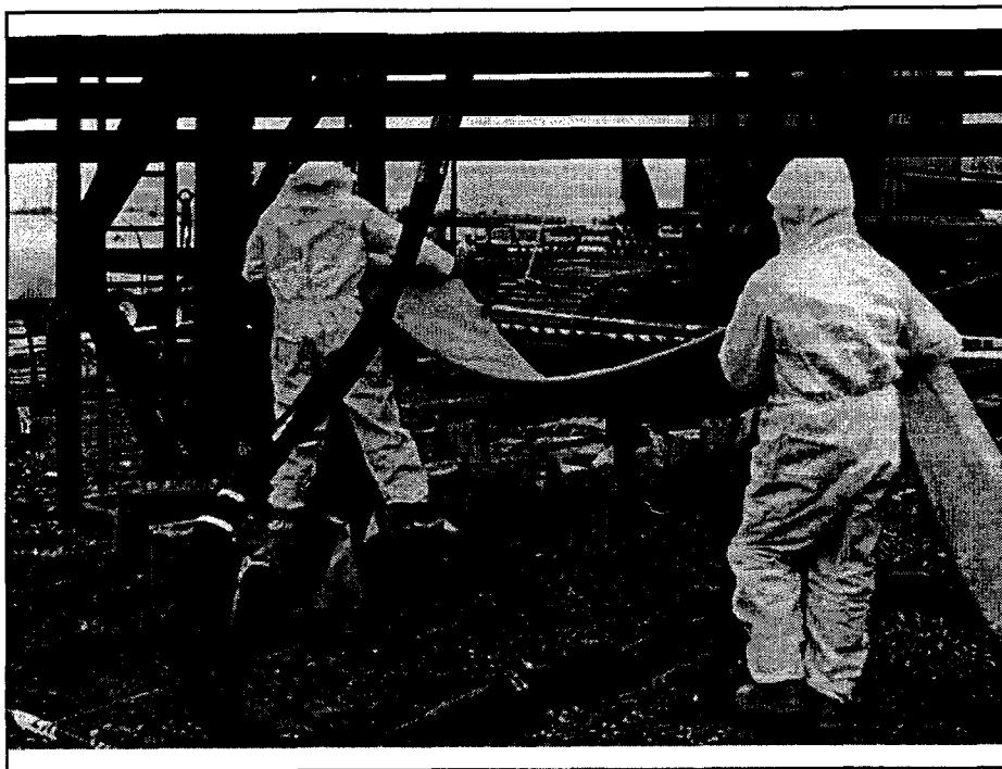
Figure 3. Wicks being installed in hollow mandrel.
