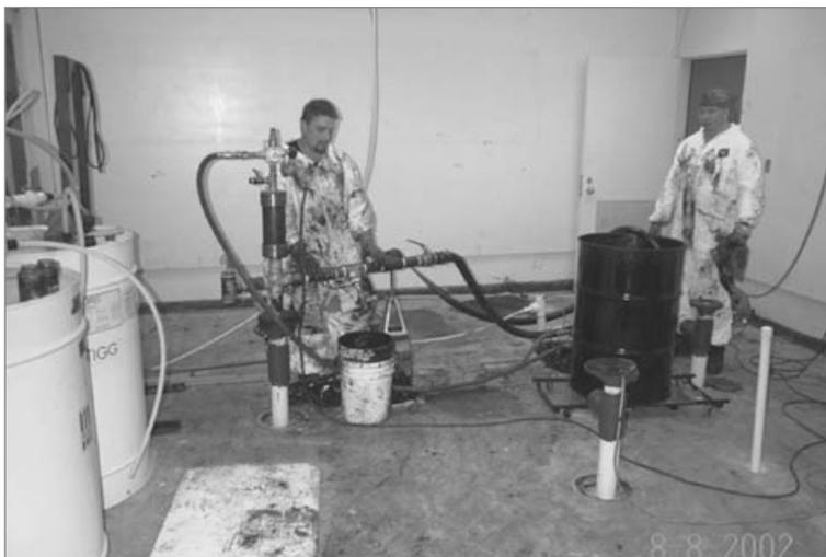
**Exhibit 3.** EZVI injection using pressure pulse technology
