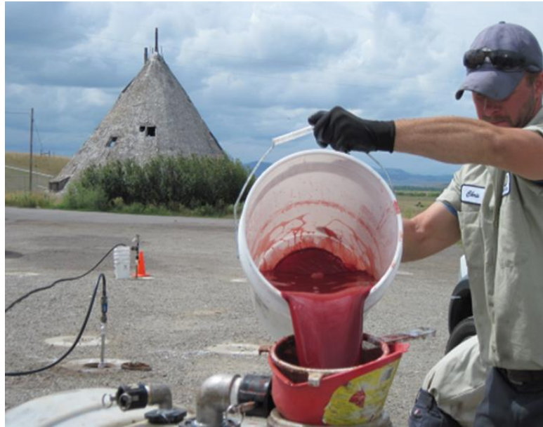
Photograph A (left) = 2% Provect-CH4 in solution with mixing. Photograph B (right) = aqueous suspension of Provect-CH4 with ca. 10% solids (some solids will settle out of suspension over time)
